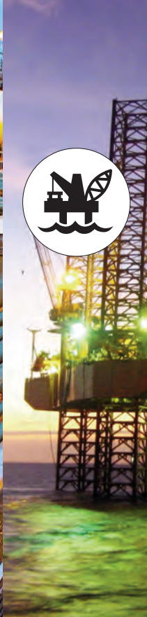
OIL PRODUCTION AND PROCESSING
