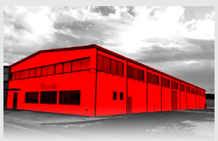
03 - Assembly & Testing plant (2.000 m 2 )
